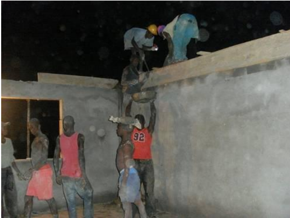
Fixing Lintel Beam
