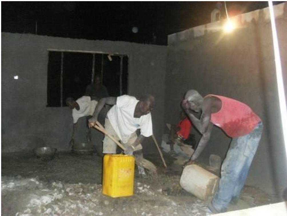
Mixing of concrete
