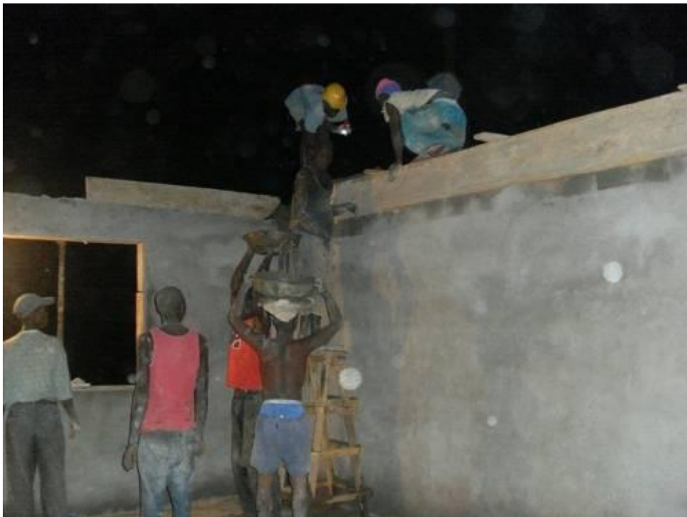
Fixing Lintel Beam
